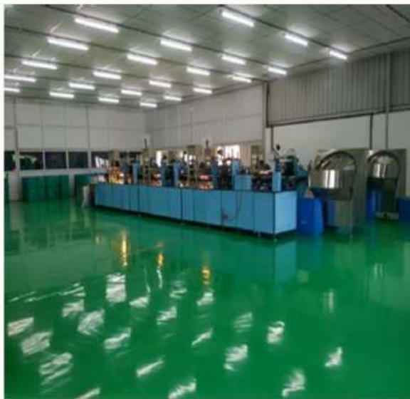
Fig.2.15 Epoxy and smooth flooring in operation, easy for cleaning and avoids dust and microbial contamination
