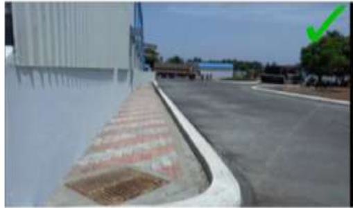
Fig.2.2 Premises with tarred and concrete to avoid dust
