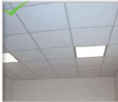
Fig.2.10 Ceiling made of impervious material
