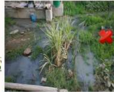
Fig.2.6 Stagnant water near the surroundings
