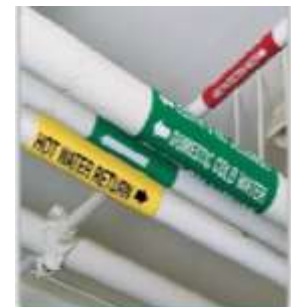
Fig.2.24 Colour coding of water pipes to avoid contamination
