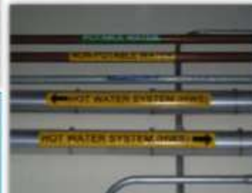
Fig.2.24 Colour coding of water pipes to avoid contamination
